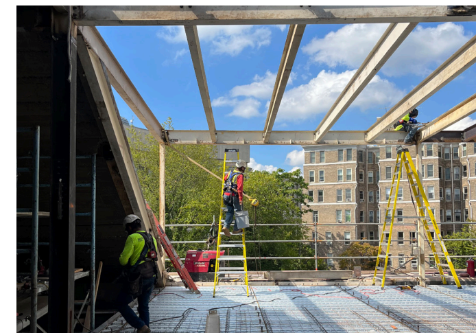
August 2024 South framing erected & floor decking installed
