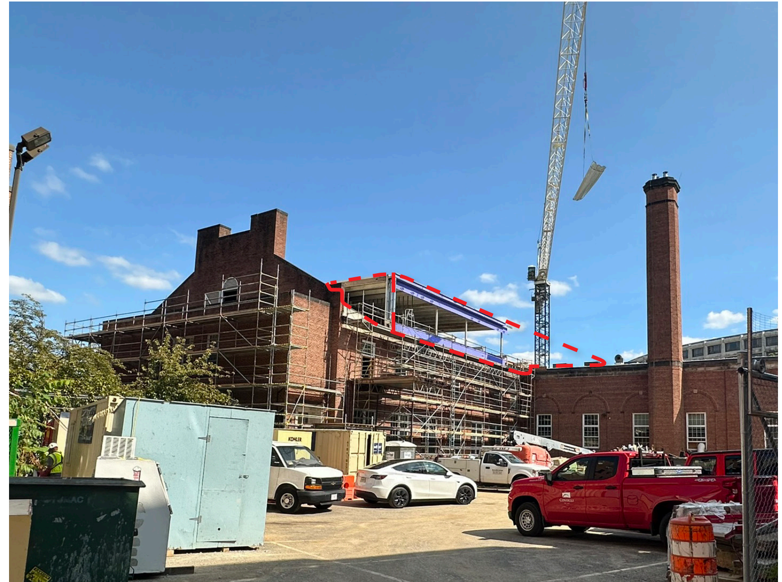
Rear, During Installation of Dormer
