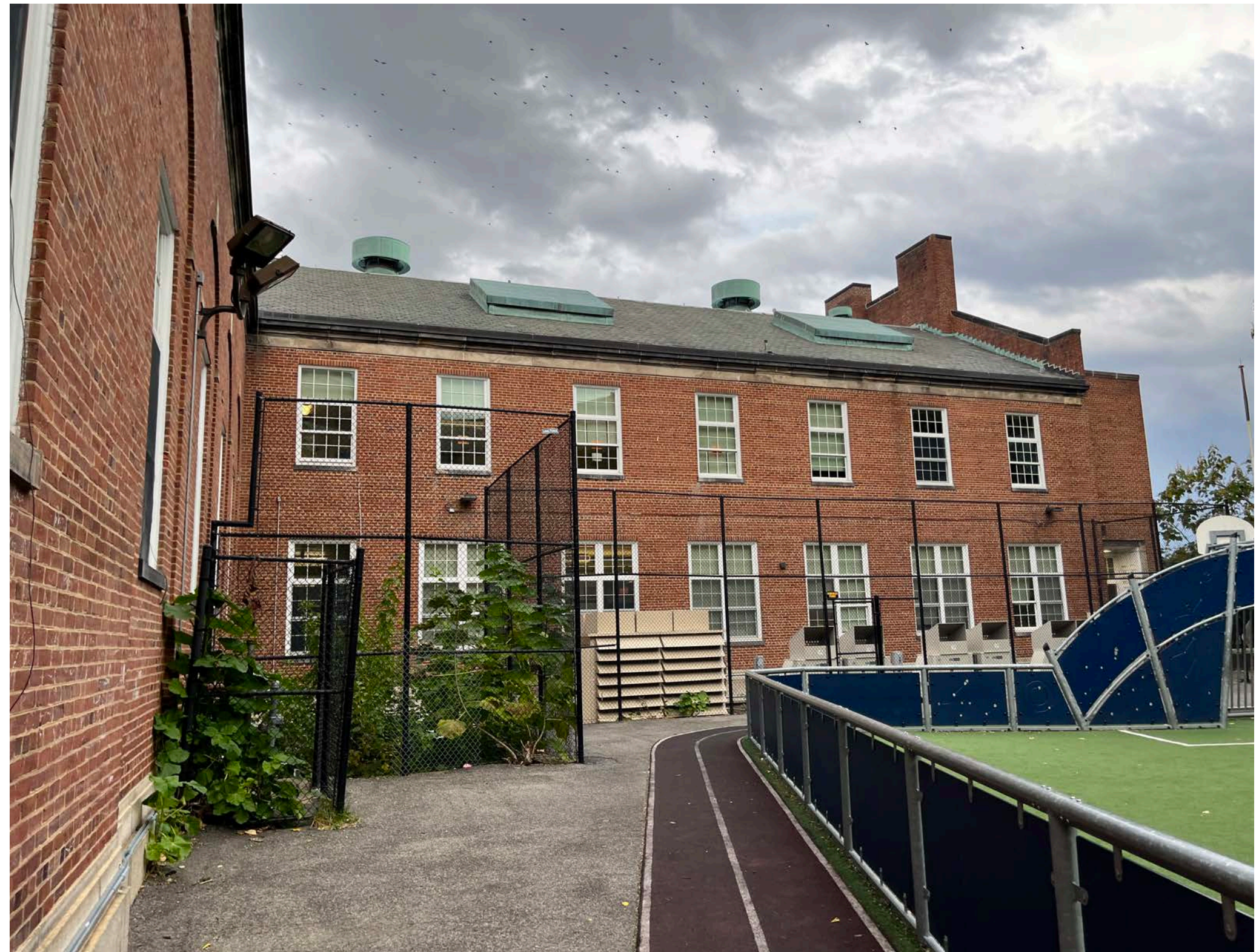
Previous Rear Facade
