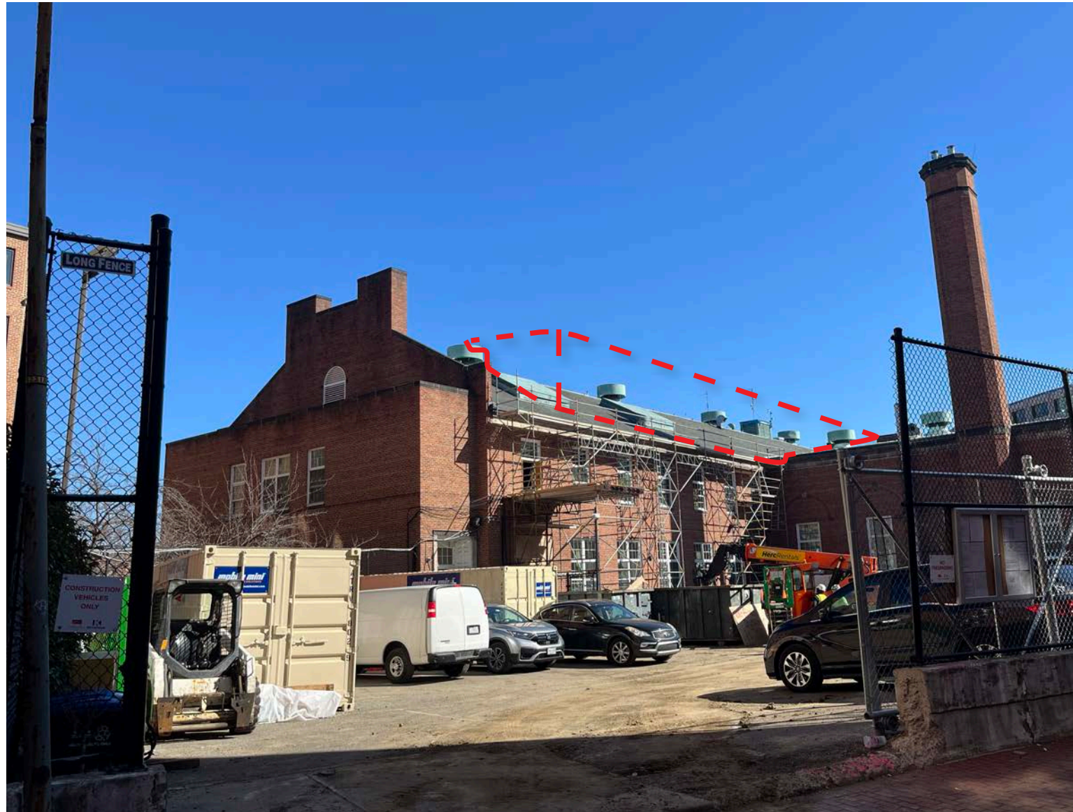
Rear, Before Roof Demo
