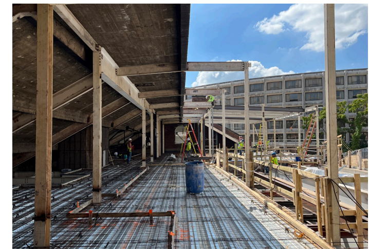
August 2024 North framing erected & floor decking
