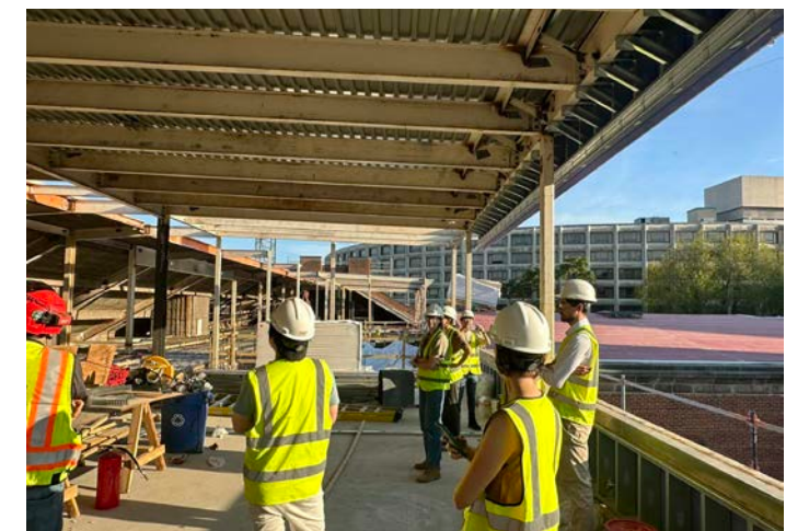
September 2024 New dormer roof decking installed
