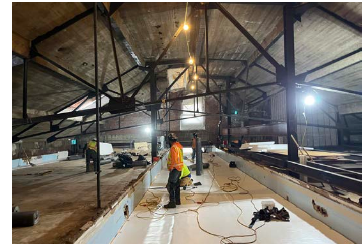
March 2024 Catch deck installation
